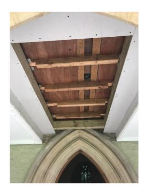
The next picture is looking up again but in the other direction and you can see the arch is exposed again on the entrance into the Nave. The frame of the lantern unit has been made and I'll have pictures of that next week. With the ceiling lifted at the entrance into the Nave, to allow the whole of the arches in the doorways to be exposed, together with glass panels above, to let more light into the Porch, there will be a much more fitting entrance into the Church.
